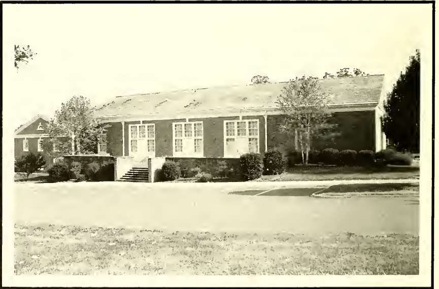
Central Hall and Administrative Wing, 1969
