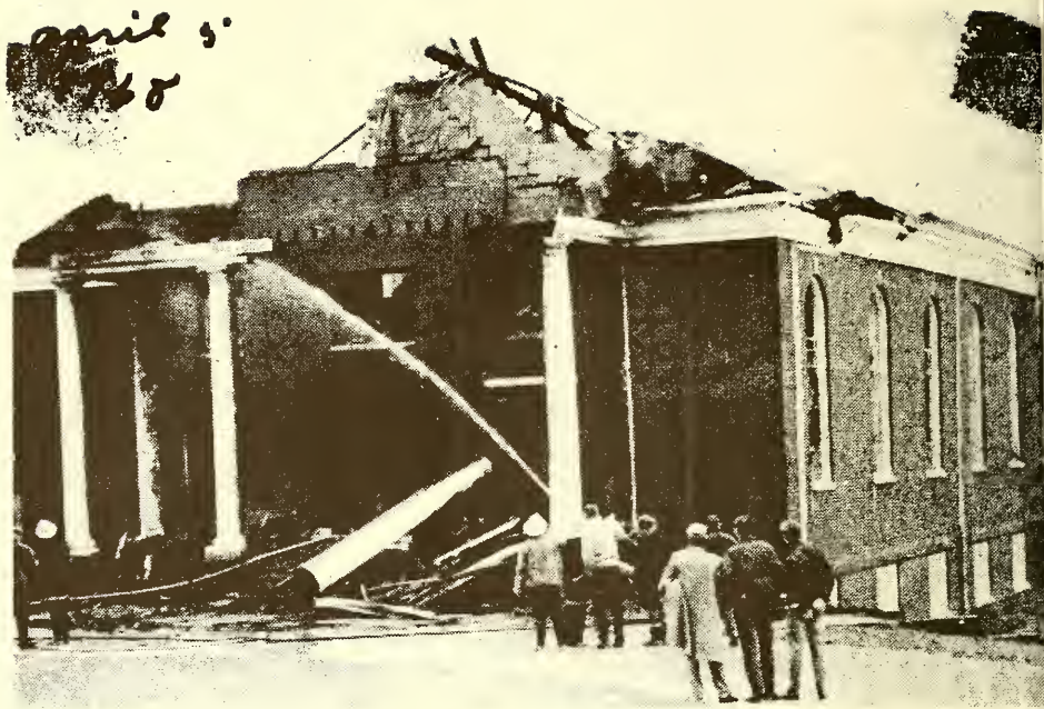
AN OUTSIDE VIEW of the Balfour Baptist Church shows the front of the church which held the steeple. Early arrivers at
