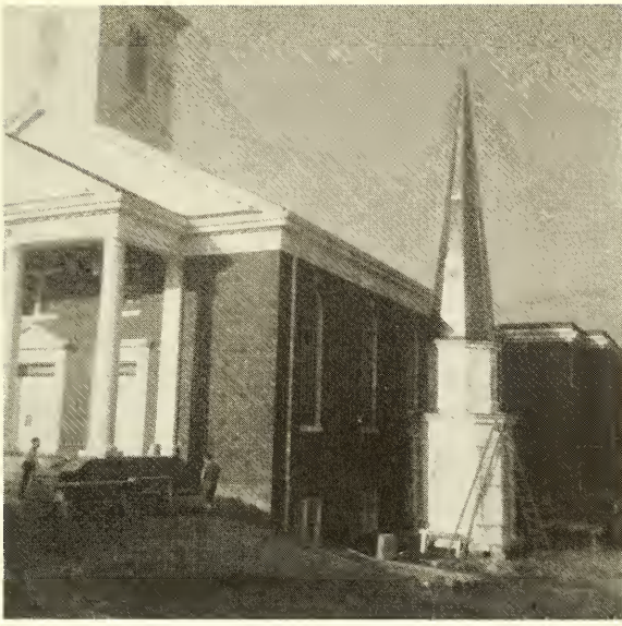
STEEPLE BEING prepared to be mounted on the new church.
