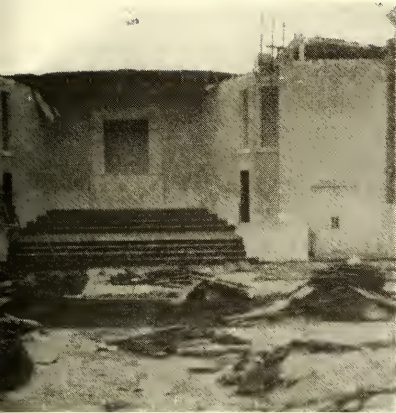
VIEW of the choir section after the fire.
