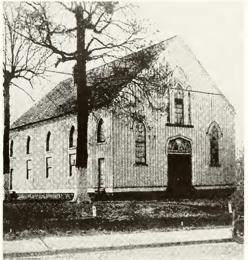
TOISNOT (WILSON, NORTH CAROLINA) PRIMITIVE BAPTIST CHURCH (MEETING-HOUSE), located at the corner of West Tarboro and Barnes Streets, where the Centre Brick Tobacco Warehouse now stands, "was the oldest church in Wilson, established in 1756." This building was used from 1859 to 1920, when it was replaced and moved to another location. It was in this building, when filled to capacity, that the Elder told Col. Bill Dortch from the pulpit, "I see Col. Bill Dortch here today. He is the brainiest lawyer in North Carolina, but he hain't got no more religion than my old mule." Elder P. D. Gold served this church as pastor from 1870 to 1920, a period of 50 years. "Toisnot" was a word from the Tuscarora Indian language, a tribe that lived nearby, meaning "a stream of water."
