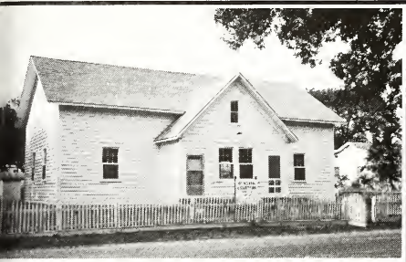
Exterior of Hunting Quarters Meeting House
