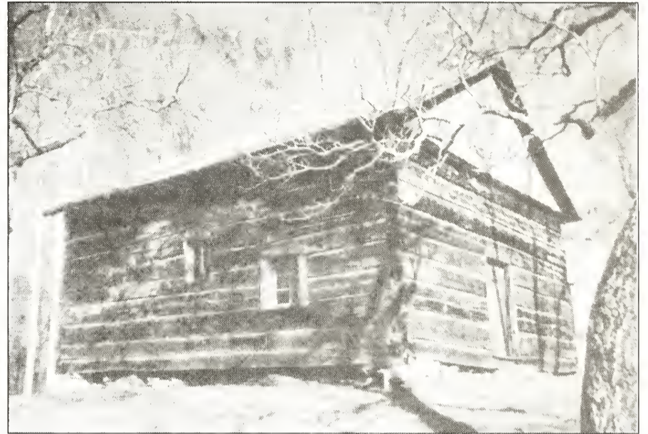
OLD SANDY CREEK PRIMITIVE BAPTIST CHURCH (LOG MEETING HOUSE), BUILT ABOUT THE YEAR 1802. SEPARATE BAPTIST PRIOR TO 1775. CHURCH FORMALLY ORGANIZED NOVEMBER 22, 1755, BY ELDER SHUBAL STEARNS. THE ABOVE 1802 STRUCTURE REPLACED THE FIRST 1762 ONE THAT WAS DESTROYED BY FIRE.
