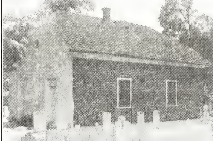
WELSH TRACT PARTICULAR BAPTIST CHURCH (MEETING HOUSE) Newark, New Castle County, Delaware
