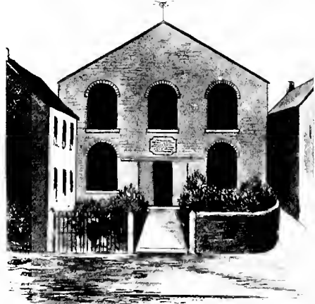
THE OLD CHAPEL AND PREACHER’S HOUSE, BEETWELL STREET, CHESTERFIELD.
