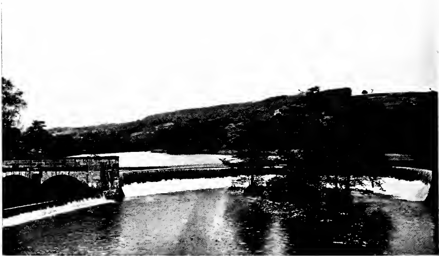
BRIDGE OVER THE DERWENT AT BELPER.
