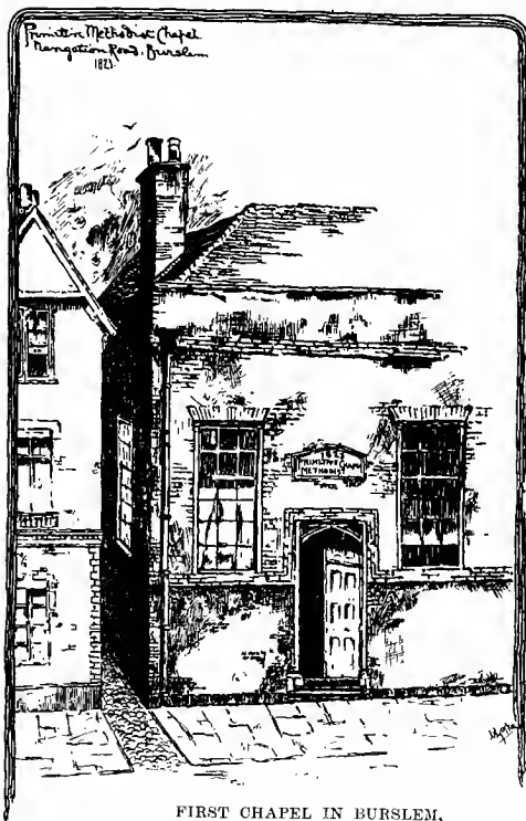
FIRST CHAPEL IN BURSLEM, As it was, now a public-house.
