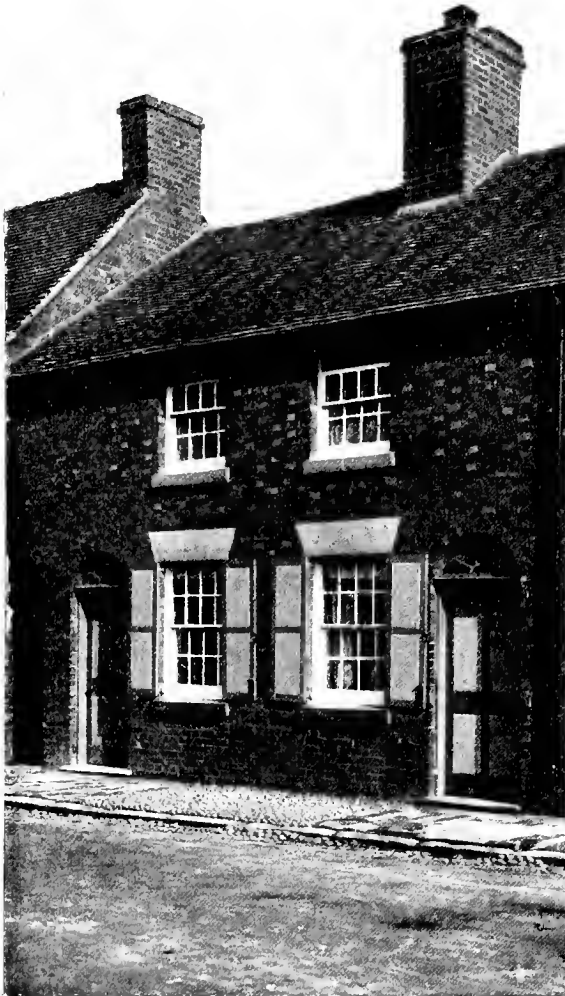
ROCESTER CHAPEL. Now turned into Two Cottages.
