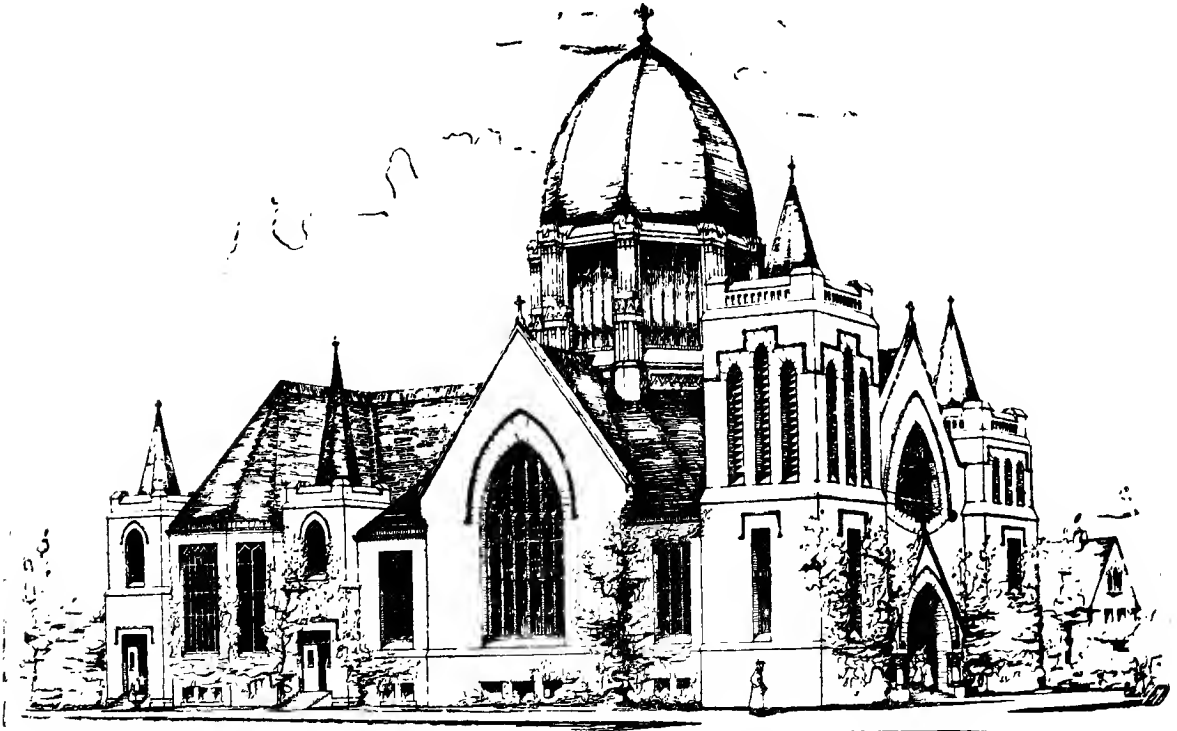
METHODIST EPISCOPAL CHURCH, WASHINGTON C. H., OHIO.
