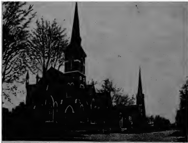
FIRST CHURCH, FREMONT. (PRESENT BUILDING.)
