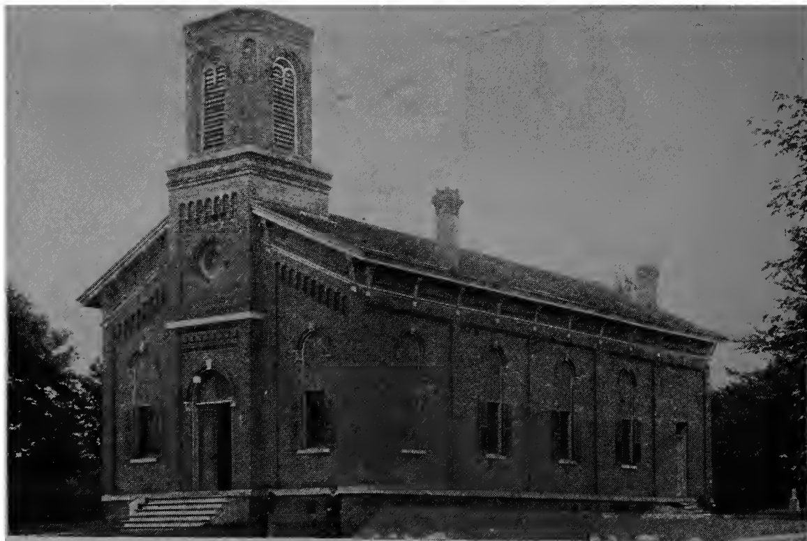
OLD COLLINGWOOD CHURCH, WEST TOLEDO. (Dismantled in 1914 for the erection of the new church.)
