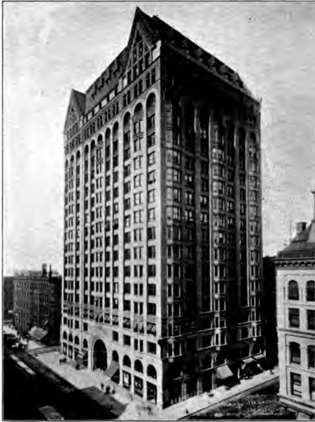
STEEL STRUCTURE—MASONIC TEMPLE, CHICAGO.
