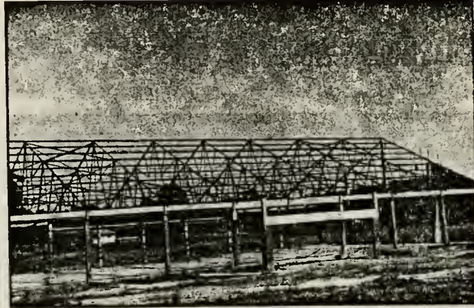
Sanctuary is now almost complete
