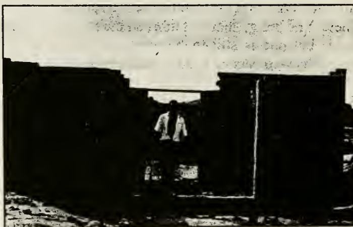
Chipfiko UMC - Sanctuary under construction
