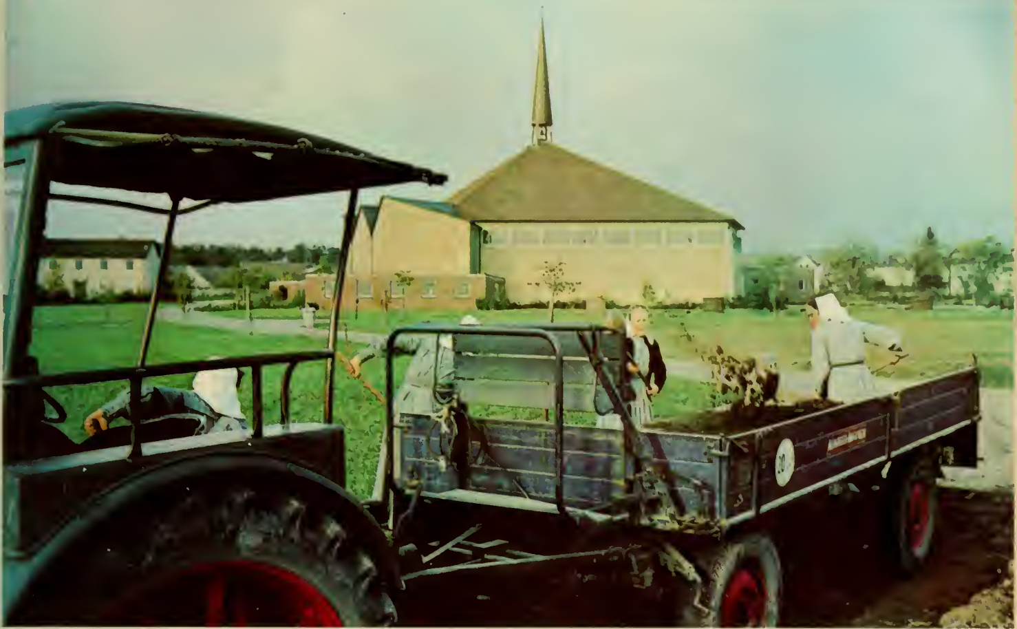
Unloading a cart, these Sisters of Darmstadt work with as much enthusiasm at building a road as they do in their continuous prayer vigil. The road leads from the community's entrance to the new Chapel of the Call of Jesus, in the background, where they present plays.
