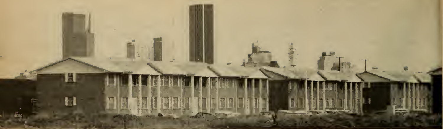
Methodist West Park Apartments stand a half mile from downtown Dallas, in an area once a slum jungle.
