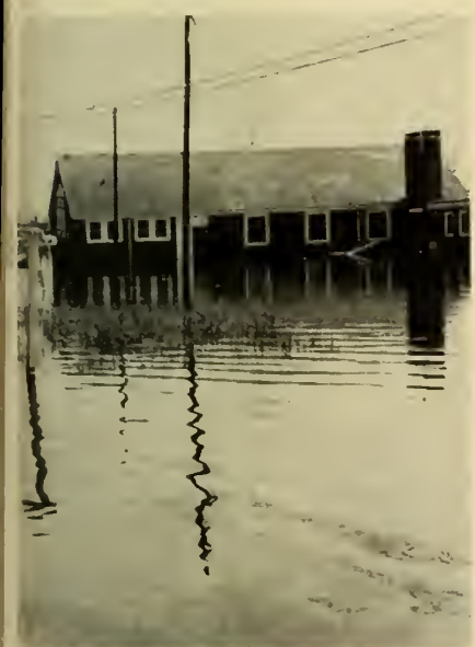
At Triumph, La., down the Mississippi River below New Orleans, flood waters stood several feet deep in Trinity Methodist Church for a full week.
