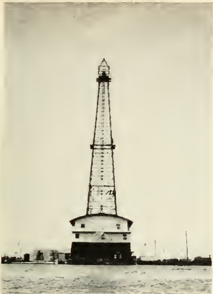
Temporary skyscraper on the Dulac horizon, this floating oil derrick soon will move out into the bayou.
