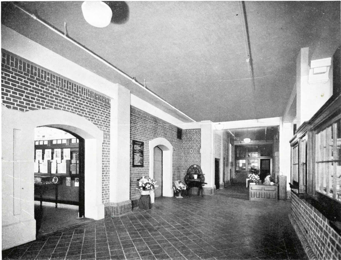
LOBBY FROM SUPERIOR AVENUE ENTRANCE
