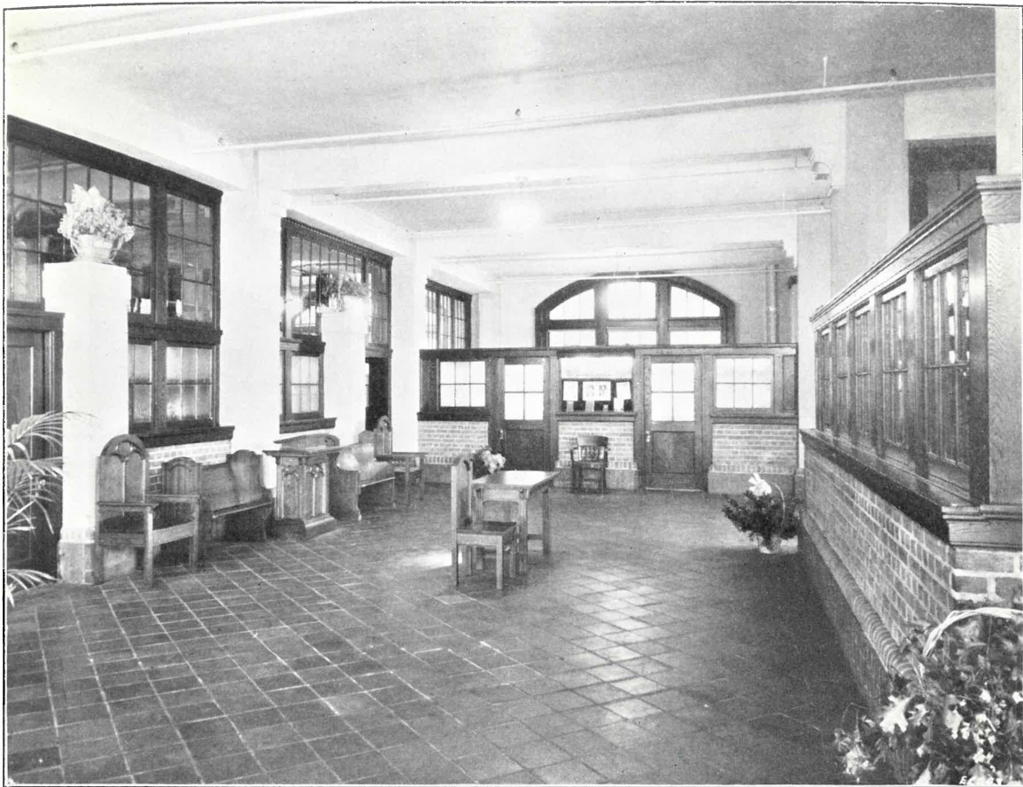
THE RIGHT WING OF THE FOYER
