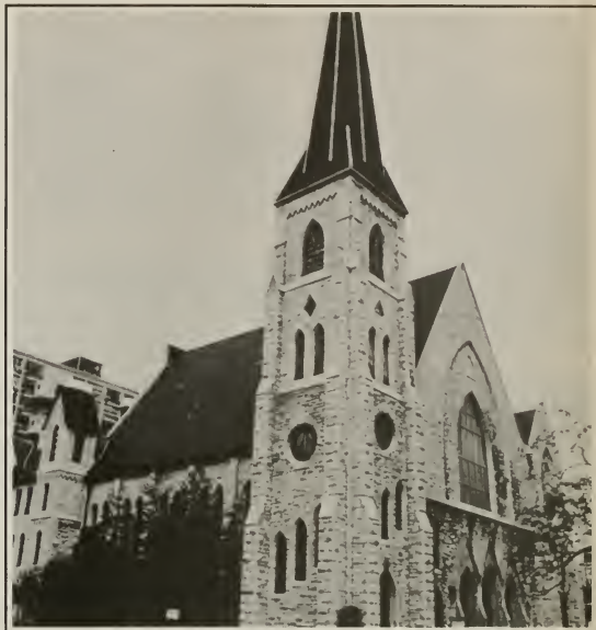
CENTENARY UNITED METHODIST CHURCH across from Union Station downtown at 16th and Pine, could be termed the Mother Church of United Methodism in St. Louis. The congregation was organized in 1839 and the present church built in 1869. The structure was one of a handful of buildings left standing when the city launched a massive urban renewal program in the late 1950s. It continues as one of the landmarks in the redeveloped area stretching from the Mississippi River through the downtown commercial district westward to Union Station.
