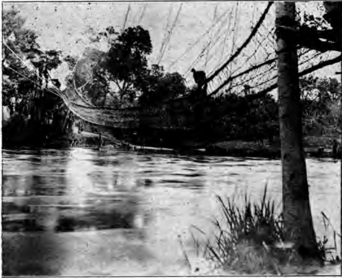
An African Suspension Bridge, Made Entirely of Vines, Across River at Lubefu Station.
