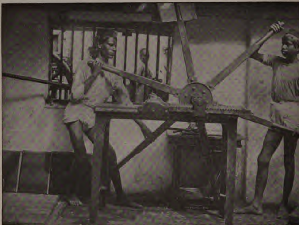
SHAVING A WAX PLATE FOR ELECTROTYPING.
