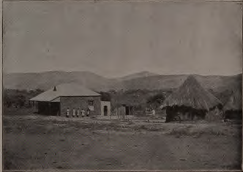
SCHOOL BUILDING AND MISSIONARY RESIDENCE, NEW UMTALI.
