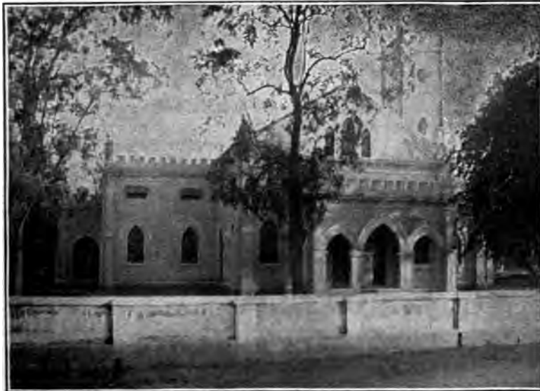
HINDUSTANI METHODIST CHURCH AT LUCKNOW.
