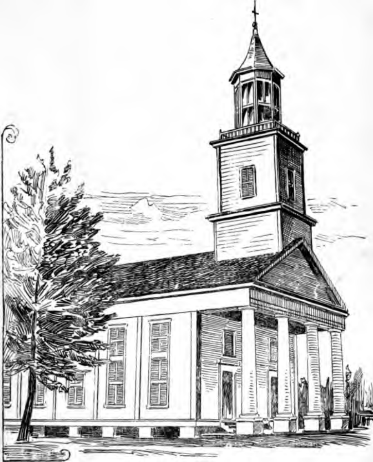
METHODIST EPISCOPAL CHURCH, SOUTH, MARION, S. C.
