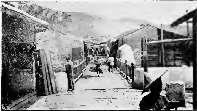
Looking along the Chaochowfu Bridge
