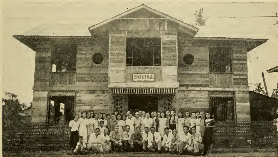
At Lingayen, Philippine Islands, a dormitory roof salvaged from a destroyed church; the fence constructed from steel runways built for planes
