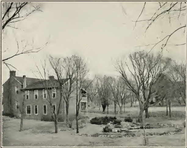
REAR OF WEST BUILDING SHOWING GARDEN POOL
