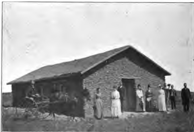
SOD METHODIST CHURCH BUILT IN TYRONE, RED WILLOW COUNTY, IN 1886. A TYPE OF MANY OF THE FIRST CHURCHES ERECTED IN NEBRASKA.
