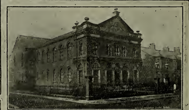
HEATON RD CHAPEL
