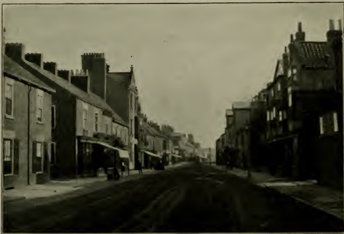
MIDDLE STREET SOUTH, DRIFFIELD.
