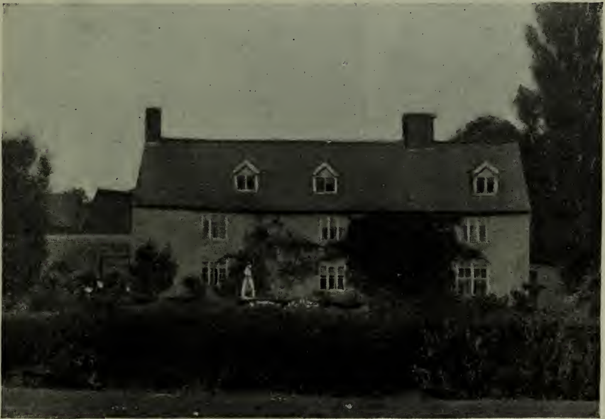
THE WOOD HOUSE, MAESBROOK.
