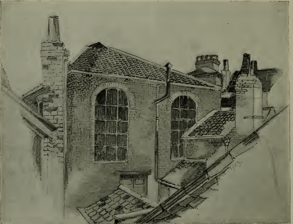
GRAPE LANE CHAPEL. THE FIRST PRIMITIVE METHODIST CHAPEL IN YORK.
