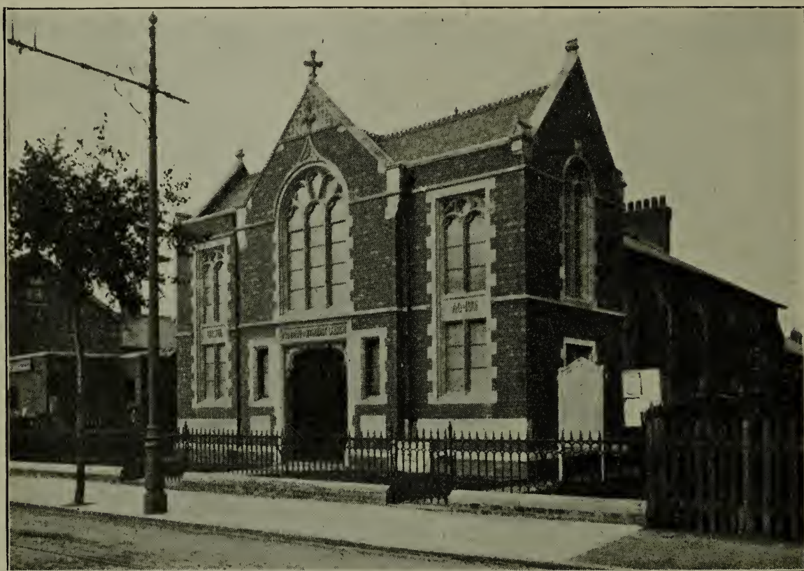
STROUD ROAD PRIMITIVE METHODIST CHAPEL, GLOUCESTER.
