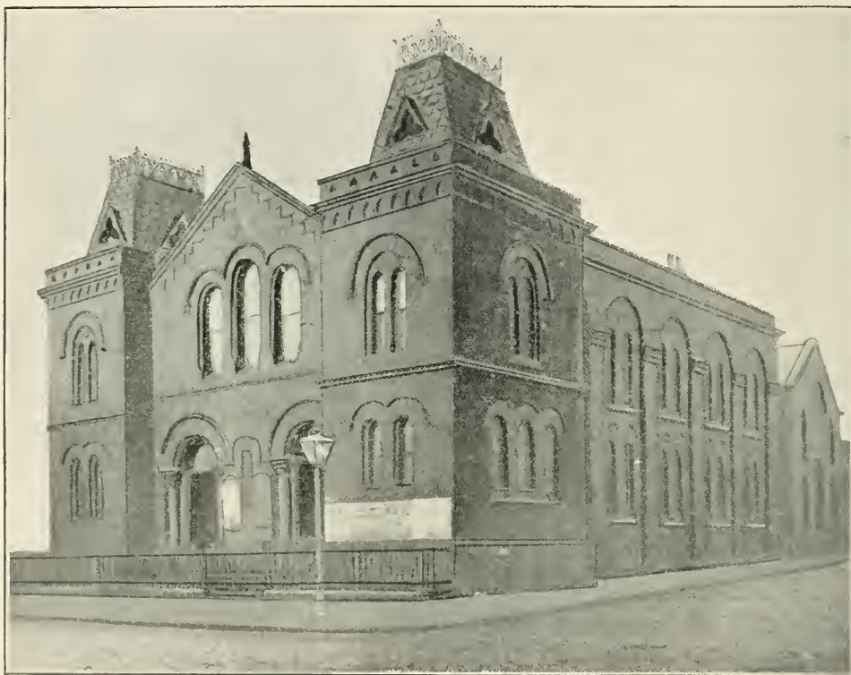
HIGHER BRIDGE STREET CHAPEL, BOLTON.
