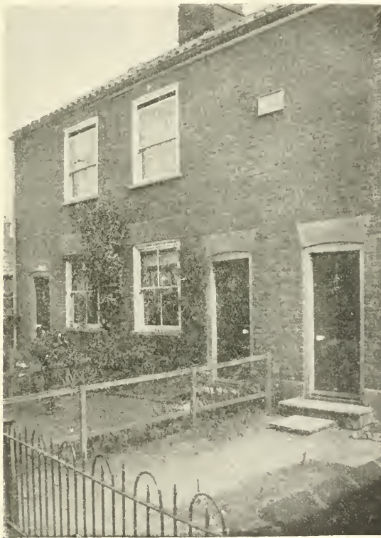
LAKENHAM OLD CHAPEL AND SCHOOL.
