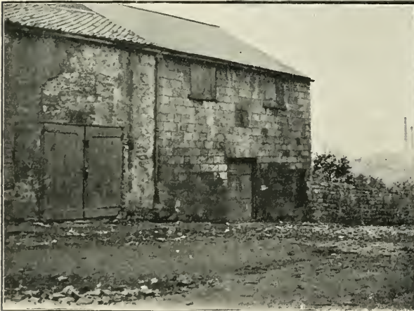
TADCASTER FIRST CHAPEL. End building, Rosemary Row.
