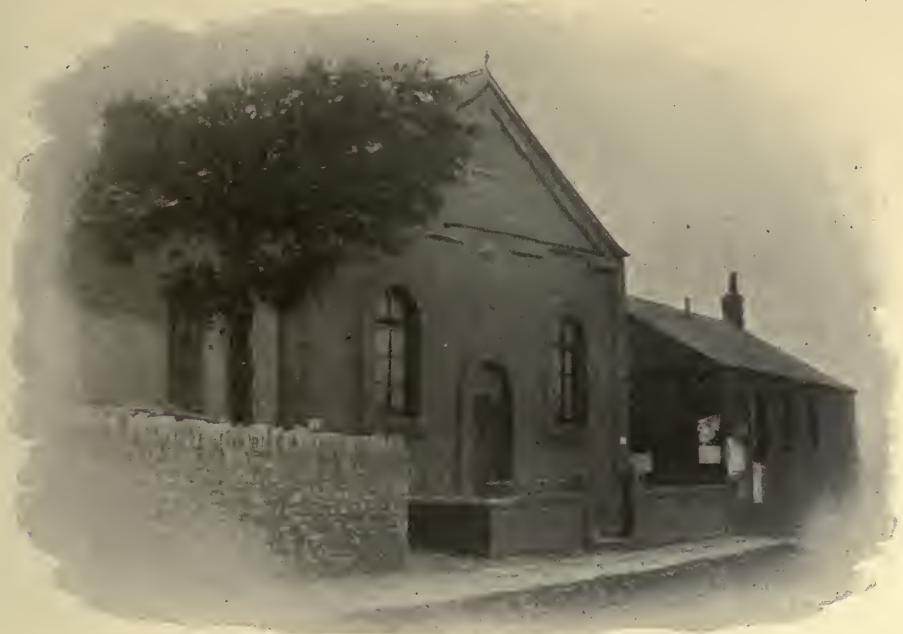
KNOTTINGLEY CHAPEL AND SCHOOLROOM, PONTEFRACT CIRCUIT.
