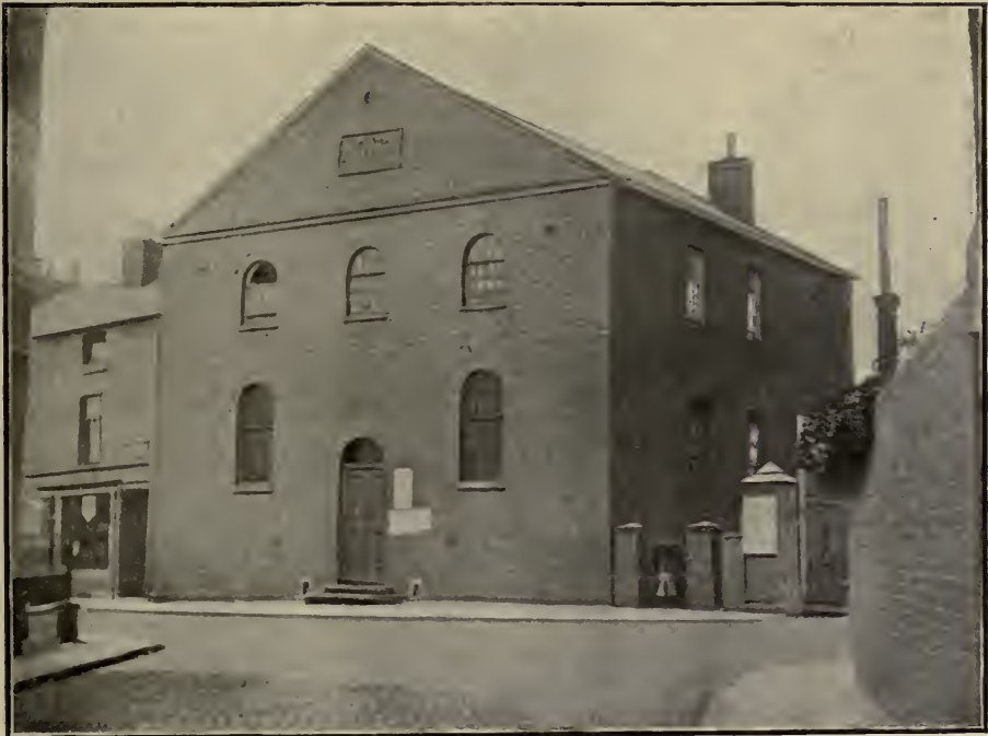
SECOND PORTLAND STREET CHAPEL.
