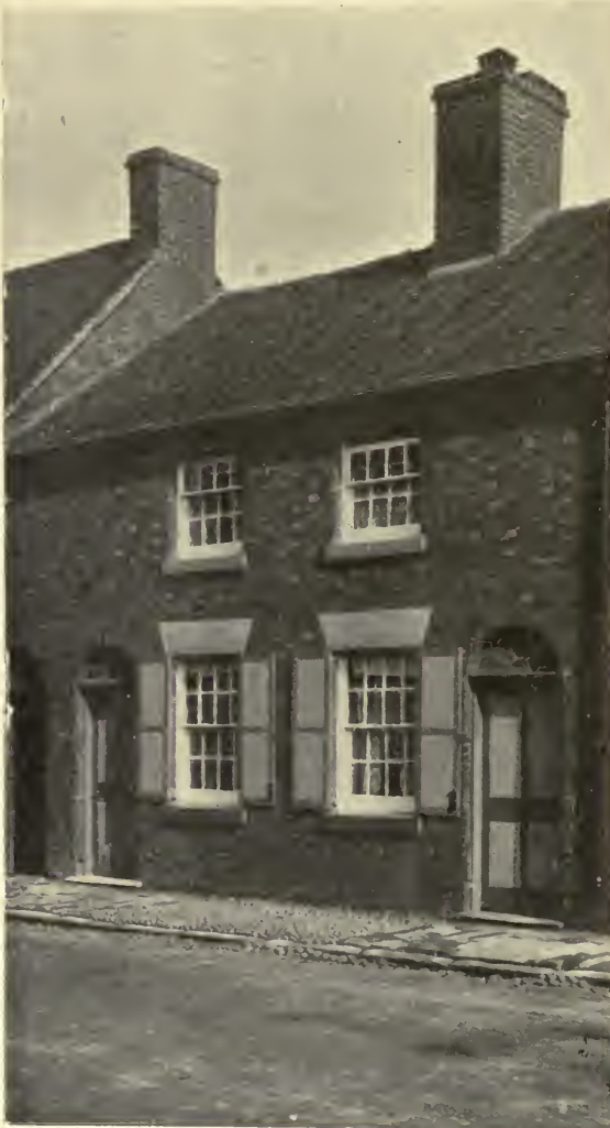
ROCESTER CHAPEL. Now turned into Two Cottages.
