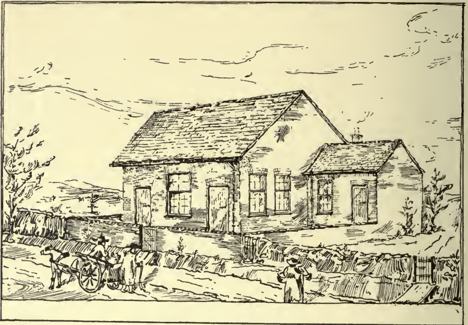
DEAD LANE PRIMITIVE METHODIST CHAPEL, LOUGHBOROUGH. 1818—1837.
