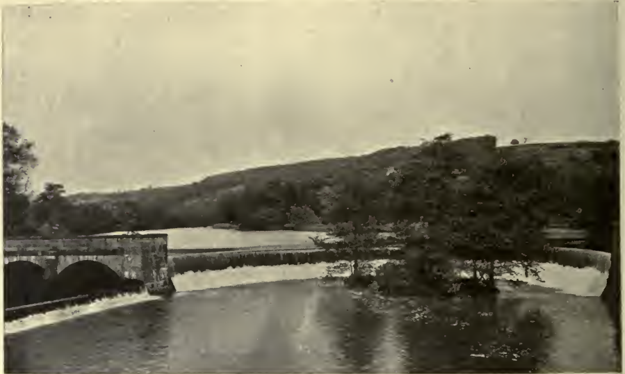
BRIDGE OVER THE DERWENT AT BELPER.
