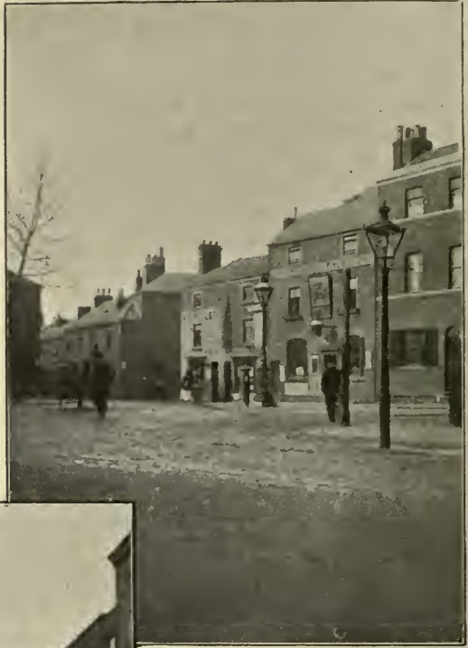
FOUNDRY SQUARE, FROM BELGRAVE GATE.
