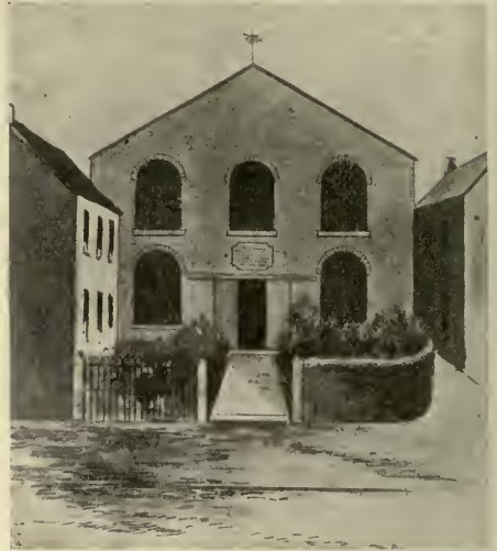
THE OLD CHAPEL AND PREACHER’S HOUSE, BEETWELL STREET, CHESTERFIELD.
