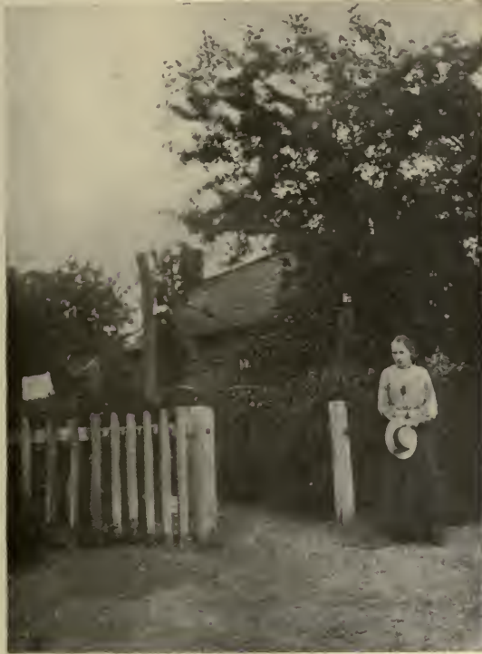
COTTAGE REBUILT ON SITE OF HENRY FUKES' HOUSE, SHELFORD.
