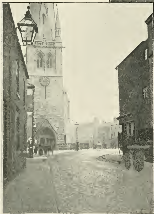
FOUNDRY SQUARE, FROM ARCHDEACON LANE.
