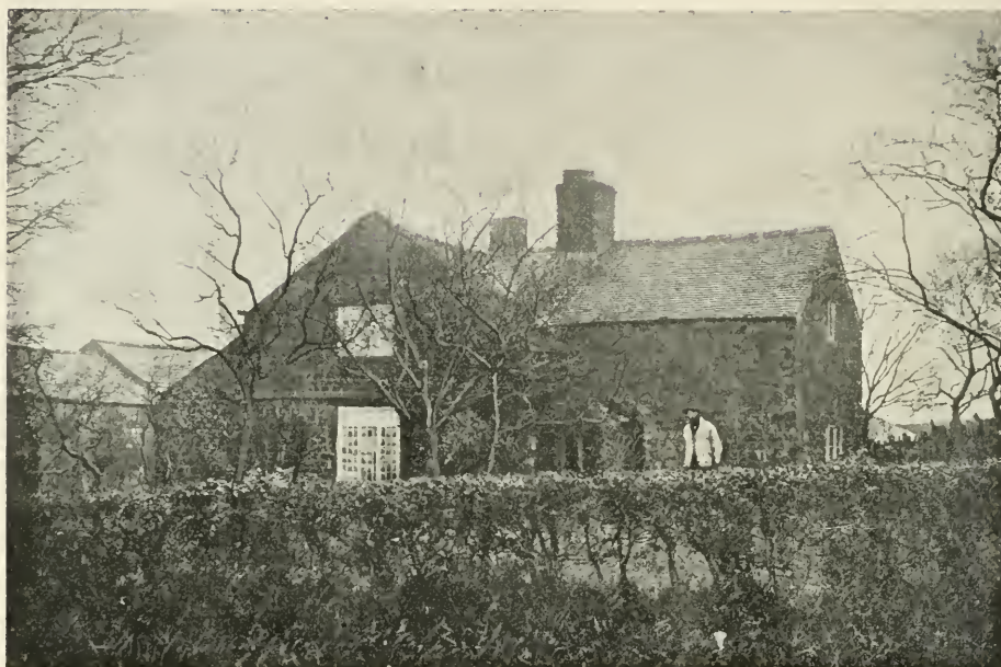
WOODHOUSE GREEN PREACHING-HOUSE. Services were held in Parlour.
