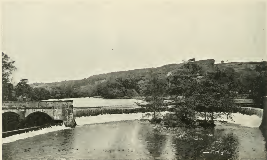
BRIDGE OVER THE DERWENT AT BELPER.
