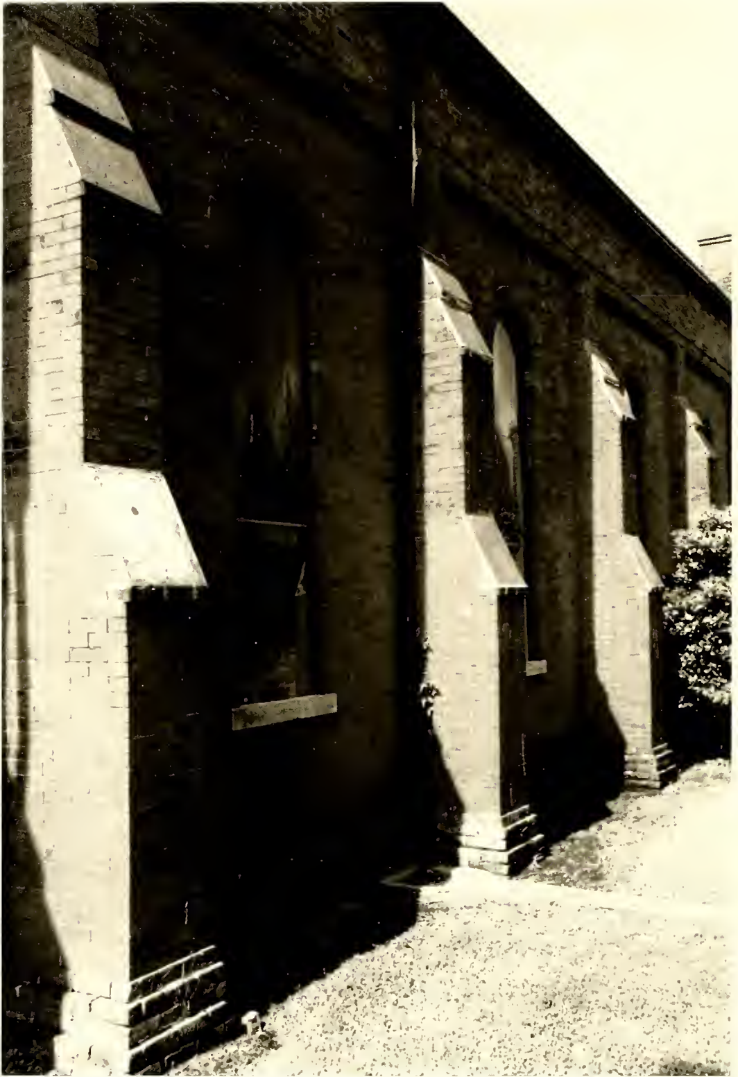
An exterior view of the Temple, facing southwest. This view shows the prominent buttresses along the sides of the auditorium, which separate the bays. This is one of the building's significant architectural design details.
