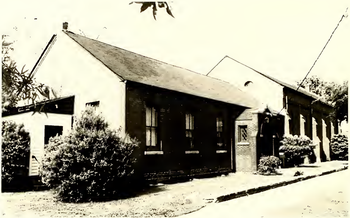
This view, facing southwest from Oak Street, shows the Sabbath school annex that was added in 1915 behind the Synagogue. There is a tiny vestibule just inside the door at center. The second door opens onto a large assembly hall.
