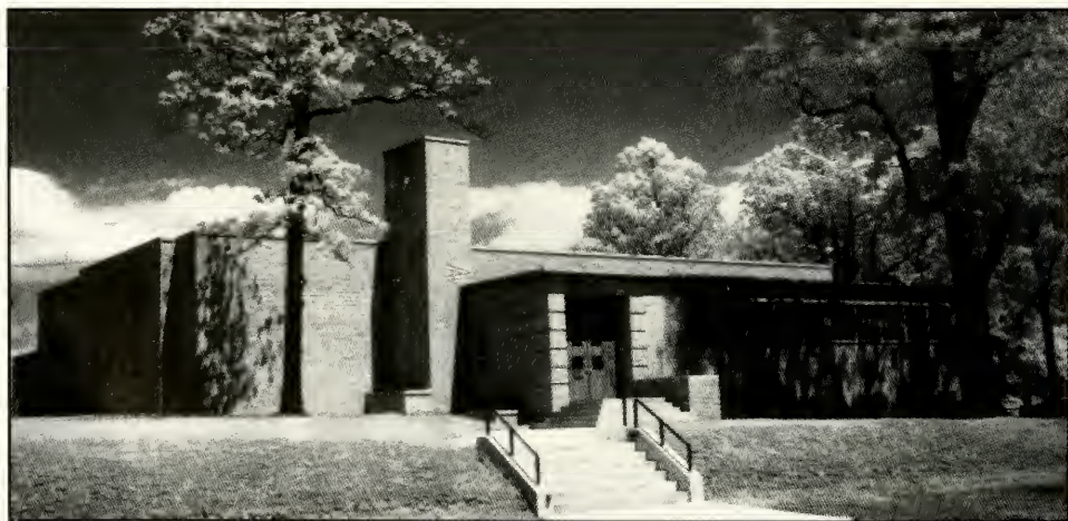
Temple Emanuel's permanent home on Oakwood Drive as it appeared in the Winston-Salem Journal in May 1952. (Forsyth County Library Photograph Collection.)
