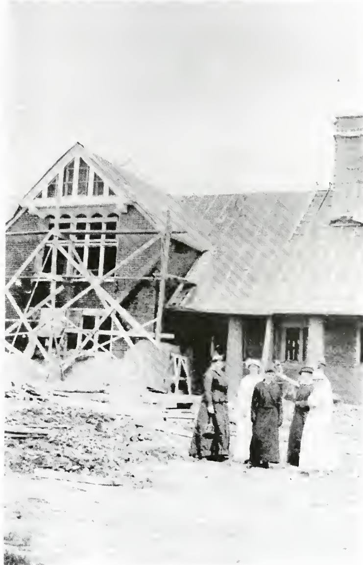
Reynolda Chapel Under Construction
