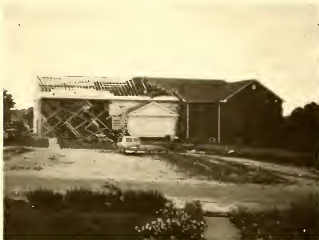
Old roof torn off and new begun.
