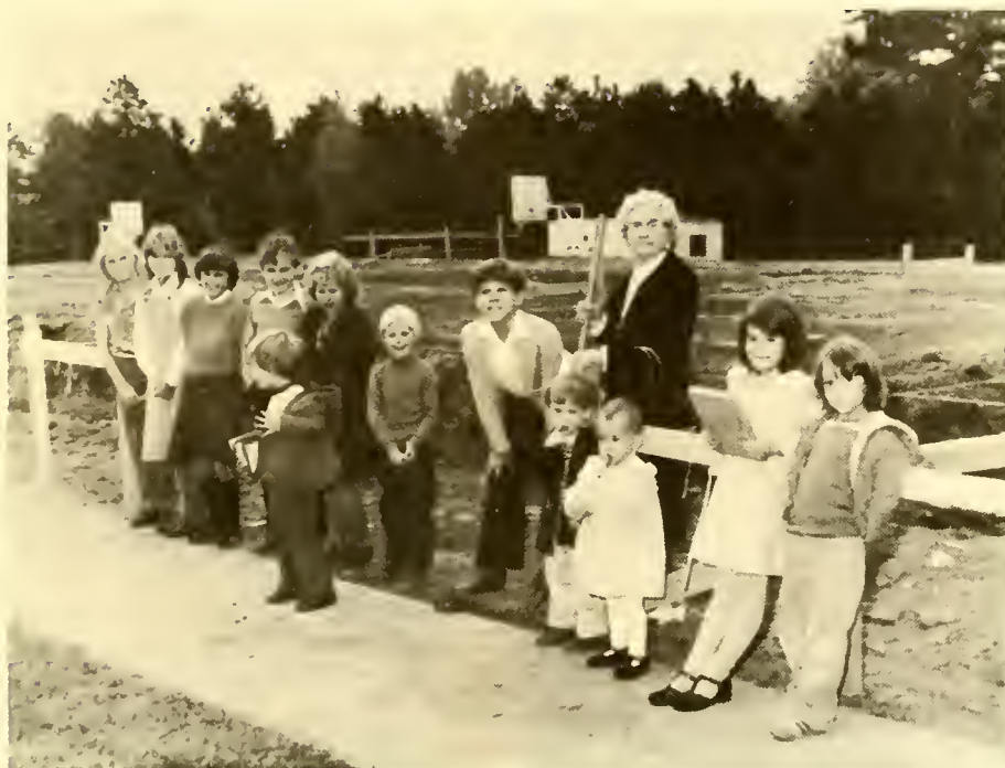
GROUND BREAKING CHURCHLAND FELLOWSHIP HALL 1980
