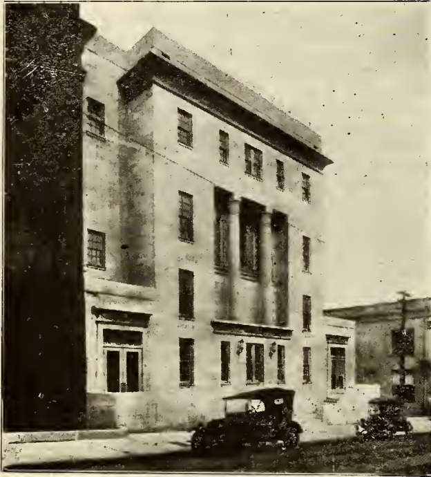
New Sunday School Building of the First Presbyterian Church, Nashville, Tenn.
