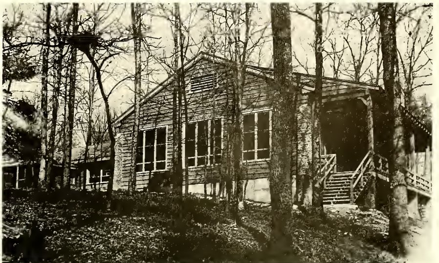
The rear of the building, showing the frame construction along with three large windows which could be easily removed when the building would be totally completed.
