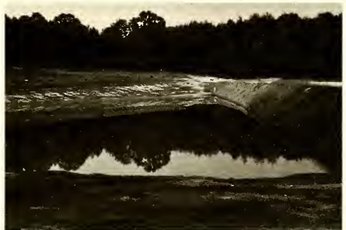
The dam completed and the basin began filling.
