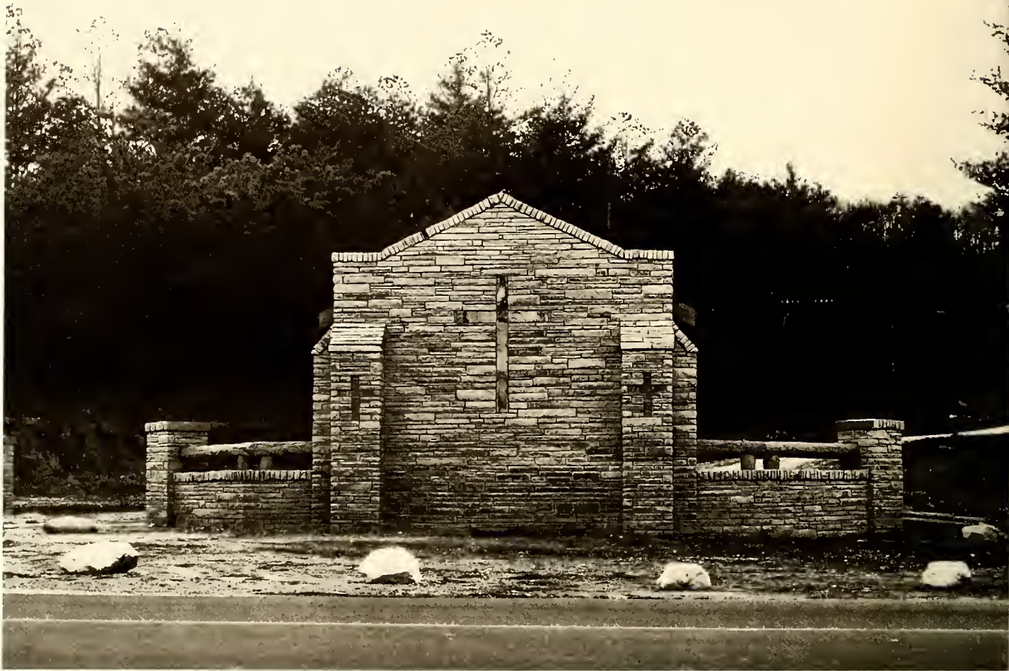
The attractive Main Entrance Gate, of wood and stone, is completed. This project was made possible through contributions of campers and other interested friends during the summers of 1953 and 1954. May all those who enter find rich blessings in Christian Community Living. The wrought iron gates were given by Mr. and Mrs. J.E. Fisher, Granite Quarry, N.C.
