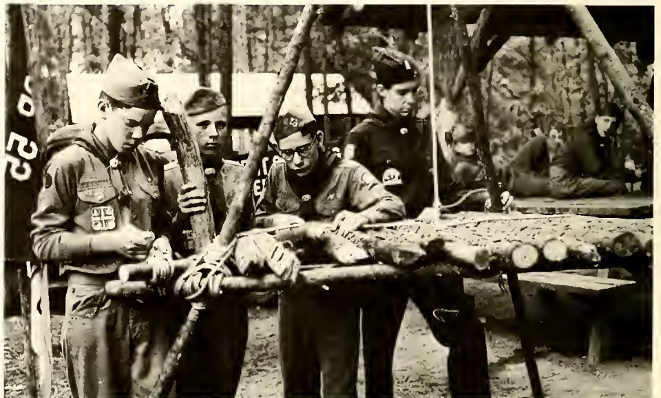
Building a signal tower.
