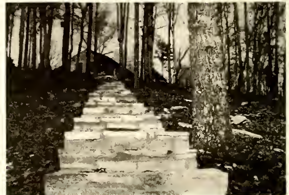
Stone steps leading from Efir Hall to the Rec. Hall.
