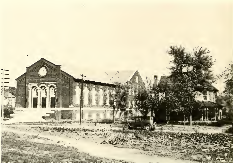
Church Sanctuary 1930 - Church Parsonage 1911- 1951
