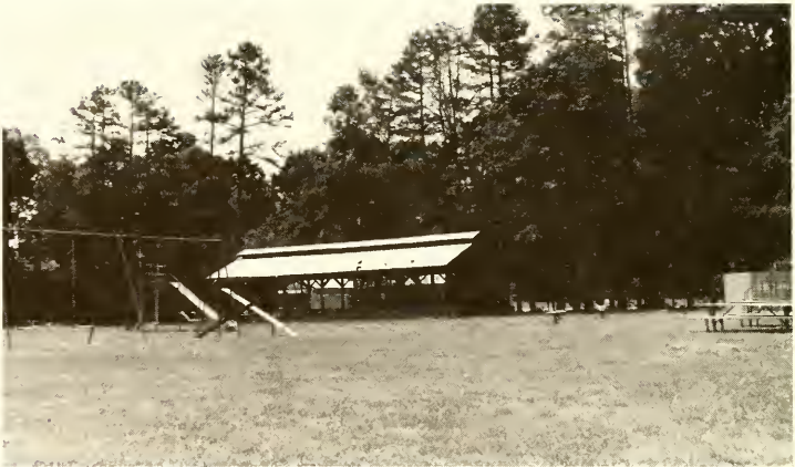
Figure 12.2 Children's and picnic area of recreation facilities with barbecue pit in background
