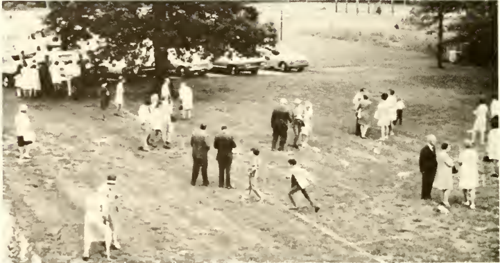
Figure 3.2 Photo showing location stakes and pipelines for new Fellowship Hall
